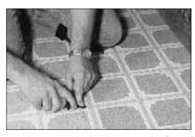
Gently squeeze the bottle to start the flow of the sealer. In a slow, continuous motion, pull the applicator along the length of the seam. The correct angle of the applicator tip to the seam is determined by the flat support or "landing face" of the VST. Most importantly, once the tip is inserted into the seam cut, it does not need to be removed until the seam is sealed, ensuring complete sealer application along the entire length of the seam.
