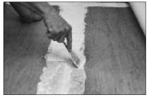
After applying the adhesive down the seam lengthwise, scrape the adhesive in the other direction (perpendicular). This will help prevent having too much adhesive in the seam. Allow the adhesive to tack up prior to laying down the resilient sheets.
