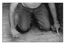
When installing 6' wide resilient flooring, snap a chalk line 6" off the wall. Also, make two additional reference marks in the center of that area. Snap a chalk line marking the center of the sheet on the floor and mark that same distance with a piece of tape on the wall.
