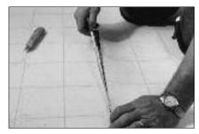
Once the seam is cut, remove the selvage edge and turn back the material to expose the subfloor.
