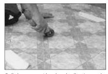
Roll the seam with a hand roller. Leave the masking tape in place to secure the seam while fitting and fastening the perimeter of the material. Also leave the masking tape in place for a minimum of one hour to allow the adhesive to set. Remove the tape just prior to seam sealing.
