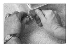
The most demanding aspect of a coved installation is forming the outside corners. Fill outside corners with a boot-type plug, rather than a V-type plug, on the least visible wall. The plugged corner fill piece should extend back at least several inches from the corner. The seam of the floor should be below the cove stick. Using an underscriber, scribe the back of the plug at the corner. This will mark the pattern of the corner on the plug.
