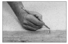
Now fit the two remaining walls, which we will name Wall A and Wall B. Make a reference mark (key mark) at the edge of the resilient sheet extending onto the subfloor with a pencil. Place a piece of tape on the long wall (the opposite edge of the sheet), visually aligning it to the pencil mark you just made on the resilient and subfloor. You will now have a reference mark on the right side of the sheet and a reference mark on the left side.
