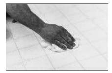
Thoroughly clean the seam area with a clean white cloth and wipe dry. Remove any adhesive that has dried on the surface with a clean white cloth dampened with a good quality-grade mineral spirits or painter's naphtha. Avoid wiping down or across the seam cut with a soiled cloth. Keep the seam cut free of soil, adhesives, or contaminants.
