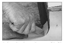
Scribe and cut the outside corners of the felt using a utility knife.
