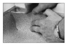
Dry fit the material. Inside corners should fit snugly, but not be forced into position. Make sure to always position the shorter side first and then the longer side. Gently pull the material away from the wall.
