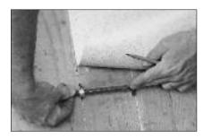
Position material squarely in room with about 2" flashed up each end of wall. Material should be positioned against the long wall overlapping the 6" reference line. Trace the edge of the sheet with a pencil marking onto the subfloor. Set dividers, or bar scriber if you need to transcribe deeper offsets, to the distance between the edge of material (pencil mark) and reference line.
