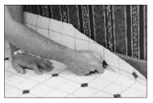
Using a sharp knife held parallel to the wall, trim away the excess material until the product is flat on the floor. Hold your cutting hand so the palm faces the wall and is out in front of you within your comfort zone. Ride the knife point at the juncture of the floor and the wall. Make sure the knife blade is flexible enough to allow some pressure to be applied to it. Hook knives and Ward type knives work well, but utility and Airway type knives do not.
