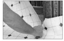
Make outside relief cuts with the floor covering held back from the corner. Cut the material from the face. You can use a pattern design line as a guide to ensure there will be sufficient material to fall around the corner.
