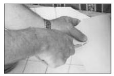
Cut a "V" when making inside relief cuts. Use your left hand to find the corner with your thumb and forefinger. Place them over floor covering into corner about 2" up the wall. Make outside relief cuts with the floor covering held back from the corner. Cut the material from the face.
