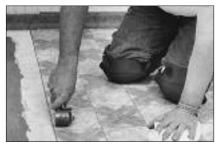
Lay one sheet into the adhesive. Roll the edge of the sheet vinyl with a hand floor roller.
