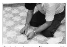
Working from the center of the seam, carefully position the second piece of resilient into alignment.
