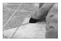
Thoroughly clean the seam cut of all adhesives, dirt, etc., before sealing the seam. It is also important to thoroughly remove any residue on the face of the material caused by the tape. Seal all seams with appropriate Mannington seam sealer (see pages 25 and 27 for directions). When inserting the VST applicator tip into the seam cut it is crucial the seam sealer be applied the full depth of the cut.
