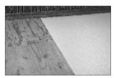
Shift the sheet back on the key marks. When the key marks are aligned, the material will fit next to Wall A. Repeat the process for the opposite wall, Wall B.
