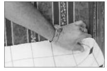
Make inside and outside corner relief cuts before trimming walls. When making any relief cuts, make them all to one side of the room first. If you need to shift floor covering, you can shift it into the cuts. If you make relief cuts on both sides of the room, when you shift the floor covering you will be short of material on one side or the other.
