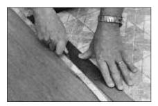
Weight the first piece of material to avoid shifting. Using a straightedge as a guide, cut the seam on one shoulder of the grout line, leaving the pattern or grout line on the sheet. When cutting seams over an existing resilient floor, protect the existing flooring from knife cuts.
