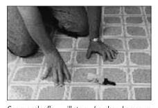
Seam sealer flow will stop when hand pressure is removed. This allows you to leave the applicator inserted in the seam cut when you reposition yourself along the length of the seam. This helps eliminate the chance of sealer skips caused by repositioning the applicator during seaming.
