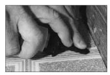
Check the flow of sealer through the applicator tip on a scrap piece of material before use. If the flow is restricted, insert the cleaning wire into the tip to clear the obstruction. Insert the plastic fin of the VST slightly back from one end of the wall and push forward to make full penetration of the fin. Use your forefinger to apply a downward pressure on the flat, textured "head" of the VST.
