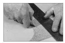
Cut along the scribed line at a 45° angle with a curved trim knife or a utility blade while holding the plug steady with a metal ruler and your other hand. When cutting, leave the face of the plug longer than the back.
