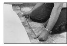
Position the material in the room, aligning the pattern squarely with the walls. Match the pattern at the seam line.
