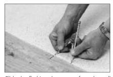
Slide the flashing sheet away from the wall (Wall A) until it lies flat on the floor and against the wall. Go back to the key mark you made on the resilient and subfloor and you will notice the mark is no longer in alignment. Set your bar scriber or dividers to that difference.
