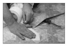
You can stretch or compress the material by using the handle of a screwdriver to bring the pattern into match. Use masking tape to hold the pattern in place on one side of the screwdriver.
