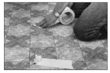
Put the seams together and place masking tape over the seam in several places to hold it in place.
