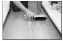
Fold back both seam edges and sweep underfloor where adhesive will be applied - the seam line and the perimeter of the room. Apply a 6" wide band of Mannington V-61 adhesive centered on the seam line.
