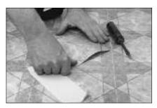
Take the screwdriver out of the seam and begin to work the seam with your hands to correctly position the design elements.
