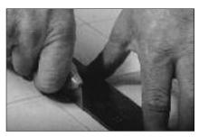
With the sheets aligned, position the steel straightedge so it completely covers the grout line of the top sheet. Using the straightedge as a guide, cut the length of the seam in the "shadow" of the grout line with a utility knife. This technique will ensure that all grout lines are of the same width. This is important, since you will completely cut away the bottom sheet grout line and will leave the grout line of the top sheet intact.
