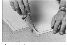
After scribing the entire work area, position sheet flooring and transcribe the pattern with pencil dividers. Be careful when cutting the material on the inside and outside corners.
