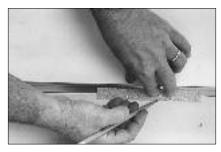
Tack the scribing felt to the wall with brad type nails before you begin to scribe it. Use a combination square, a small metal ruler, or a 1" piece of resilient to pattern scribe the felt. Fit the scribing tool up inside the cove cap and scribe the felt by sliding the tool along the cap as you mark the felt with a pencil.
