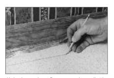
Slide the resilient flooring to the wall. The sheet should now be positioned on the 6' reference line and next to the long wall.
