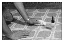
Before sealing the seam, make sure the seam cut is clean, dry, and free of adhesive contamination. Shake the seam sealer container to blend the ingredients and allow air bubbles to disperse (usually 15 minutes) before pouring sealer into the applicator bottle. Fill the bottle at least 2/3 full with the appropriate seam sealer and tightly screw on the VST applicator tip.
